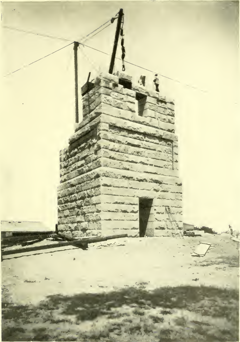
THE PILGRIM MONUMENT IN CONSTRUCTION.
